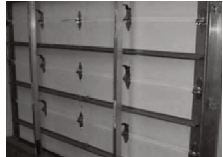
Reinforced Garage Door
