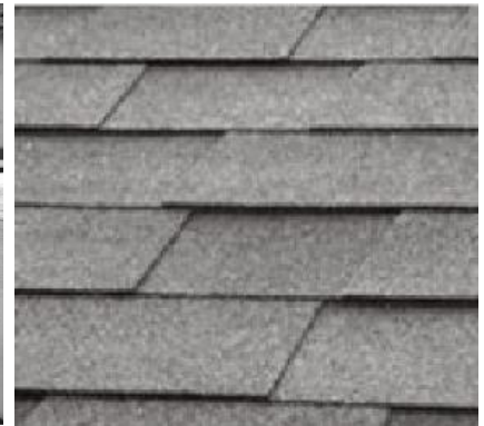
Upgrade of roof coverings
