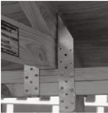
Roof to wall Connections
