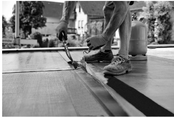
Exterior Secondary Water Barrier
